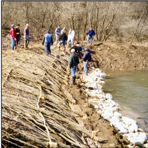
Streambank stabilization structure.
