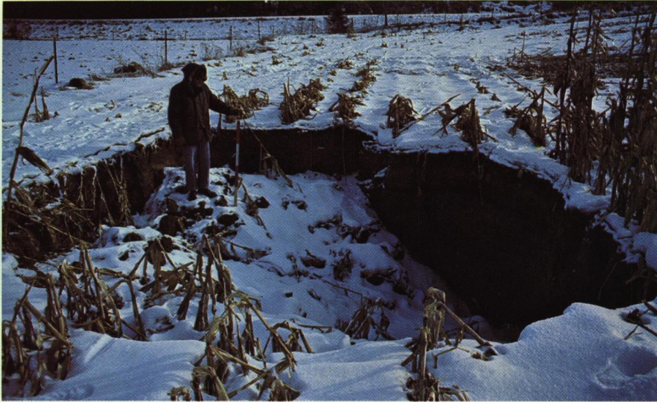
This Clayton County sinkhole opened suddenly last fall. Photo by Greg Ludvigson.
