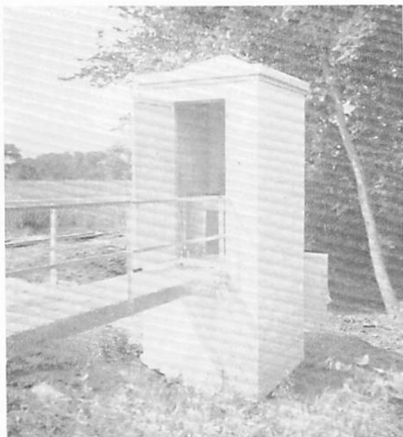
B. CONCRETE BLOCK GAGE HOUSE ON WEST FORK SHELL ROCK RIVER AT FINCHFORD, IOWA
