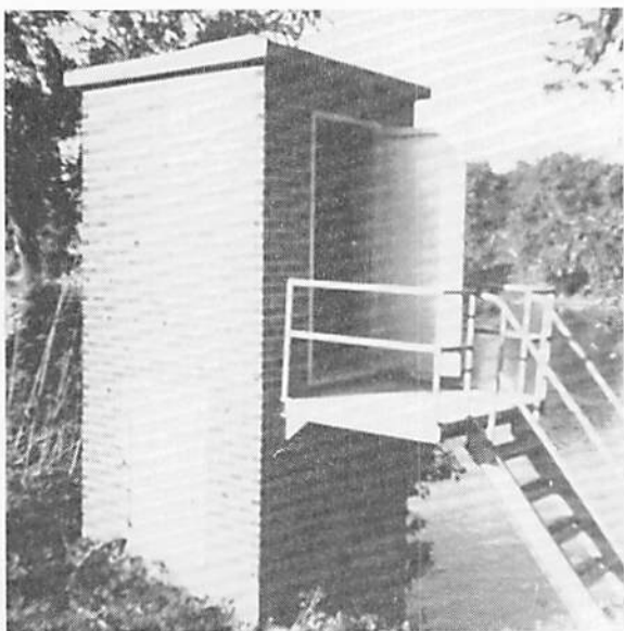
A. BRICK GAGE HOUSE AND CONCRETE WELL ON DES MOINES RIVER AT FORT DODGE, IOWA
