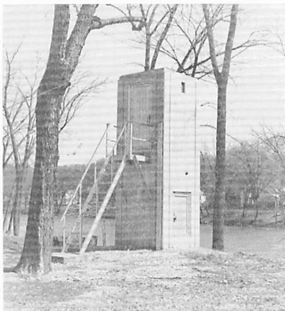
A. CONCRETE GAGE HOUSE ON WAPSIPINICON RIVER AT INDEPENDENCE, IOWA
