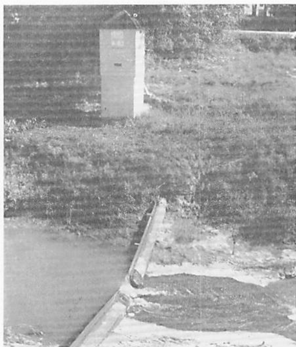
B. GAGE HOUSE AND ARTIFICIAL CONCRETE CONTROL ON RAPID CREEK NEAR IOWA CITY, IOWA
