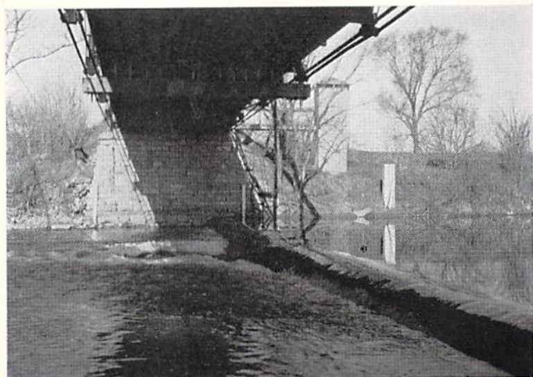
A. ARTIFICIAL CONTROL AND RECORDING GAGE INSTALLATION ON LIME CREEK AT MASON CITY, IOWA
