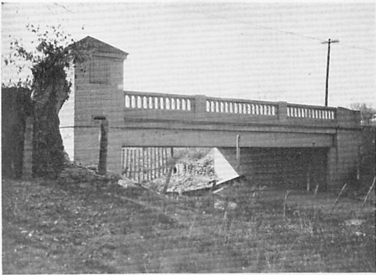
B. ARTIFICIAL CONTROL UNDER STATE HIGHWAY BRIDGE, ROUTE No. 1, AND RECORDER HOUSE ON RALSTON CREEK AT IOWA CITY, IOWA
