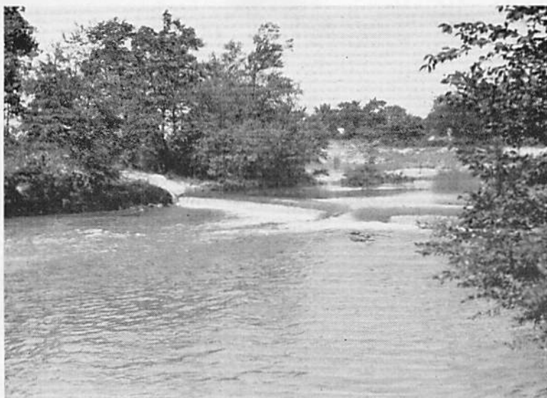
B. ARTIFICIAL CONTROL FOR GAGING STATION ON MAQUOKETA RIVER NEAR MANCHESTER, IOWA GAGING STATION EQUIPMENT
