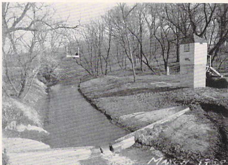
A. ARTIFICIAL CONTROL, GAGE HOUSE, AND CABLEWAY ON RAPID CREEK NEAR IOWA CITY, IOWA
