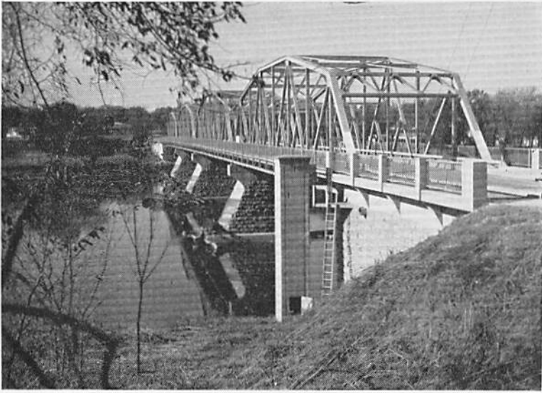
A. STATE HIGHWAY BRIDGE AND REINFORCED CONCRETE GAGE HOUSE AND WELL ON DES MOINES RIVER AT KEOSAUQUA, IOWA
