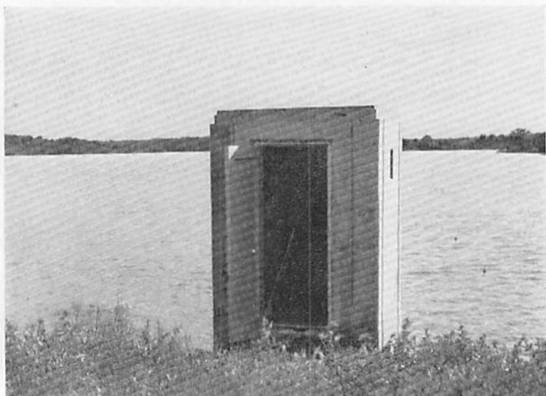
A. RECORDER HOUSE AT WATER-LEVEL GAGE ON LAKE WAPELLO NEAR DRAKESVILLE, IOWA
