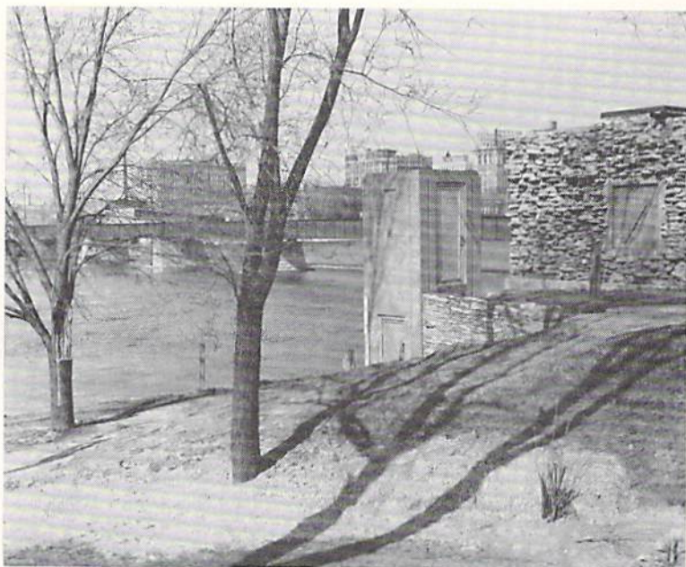
Figure 7. CONCRETE GAGE HOUSE ON CEDAR RIVER AT WATERLOO, IOWA, DURING LOW FLOW.
