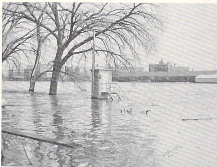
Figure 3. CONCRETE GAGE HOUSE ON CEDAR RIVER AT CEDAR RAPIDS, IOWA, AT PEAK OF FLOOD ON MARCH 31, 1961.
