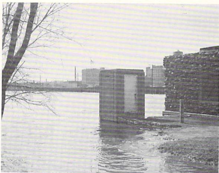
Figure 6. CONCRETE GAGE HOUSE ON CEDAR RIVER AT WATERLOO, IOWA, AT PEAK OF FLOOD ON MARCH 29, 1961.
