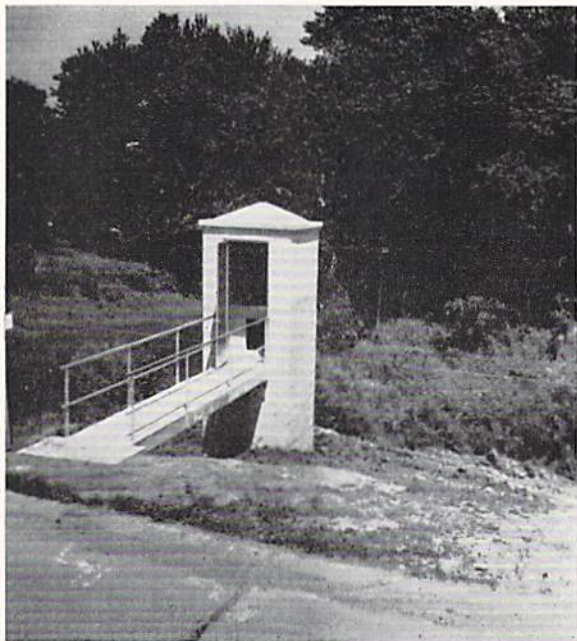
A. CONCRETE BLOCK GAGE HOUSE ON NORTH SKUNK RIVER NEAR SIGOURNEY, IOWA
