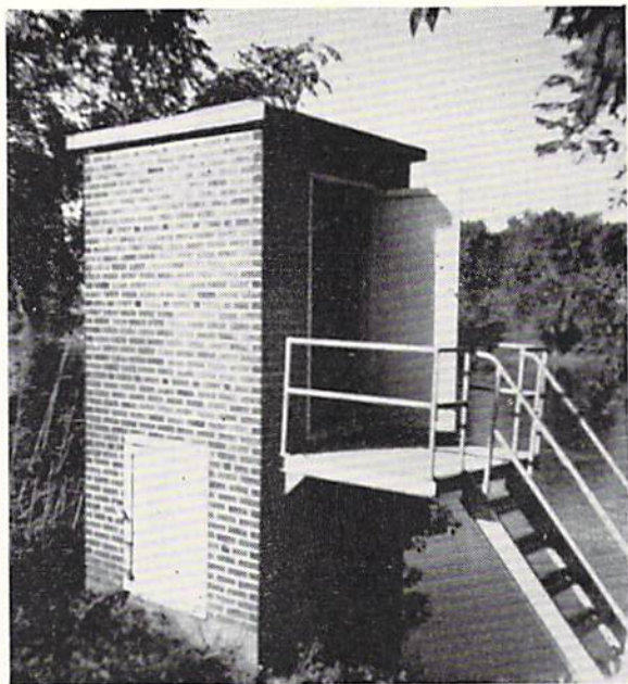
A BRICK GAGE HOUSE AND CONCRETE WELL ON DES MOINES RIVER AT FORT DODGE, IOWA
