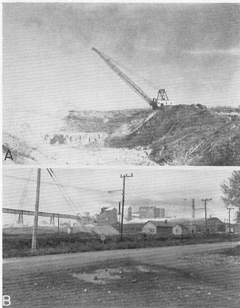
PLATE 7.—A, GYPSUM QUARRY IN THE NW¼ SEC. 26, T. 89 N., R. 28 W., SHOWING THE THICK BED OF GYPSUM AND THE SHALE AND DRIFT OVERBURDEN; B, PLANT FOR MANUFACTURING GYPSUM PRODUCTS, LOCATED NEAR FORT DODGE, IOWA.
