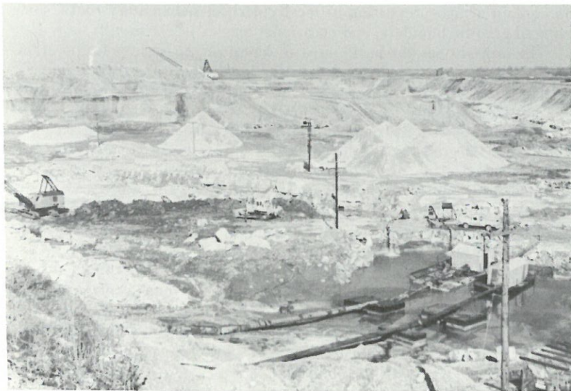
Figure 1. General view of quarry, looking northeast. Test-run production of stone has been made, and portable crusher and stacker have been removed. Sump is in right foreground, beginnings of limestone quarry in center beyond bulldozer. Dragline removing gravel is partly visible in the distance.
