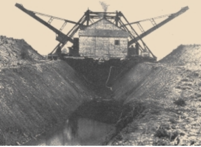
Photo from Report of the Iowa State Drainage Waterways and Conservation Commission, State of Iowa, 1911, Plate 5.
