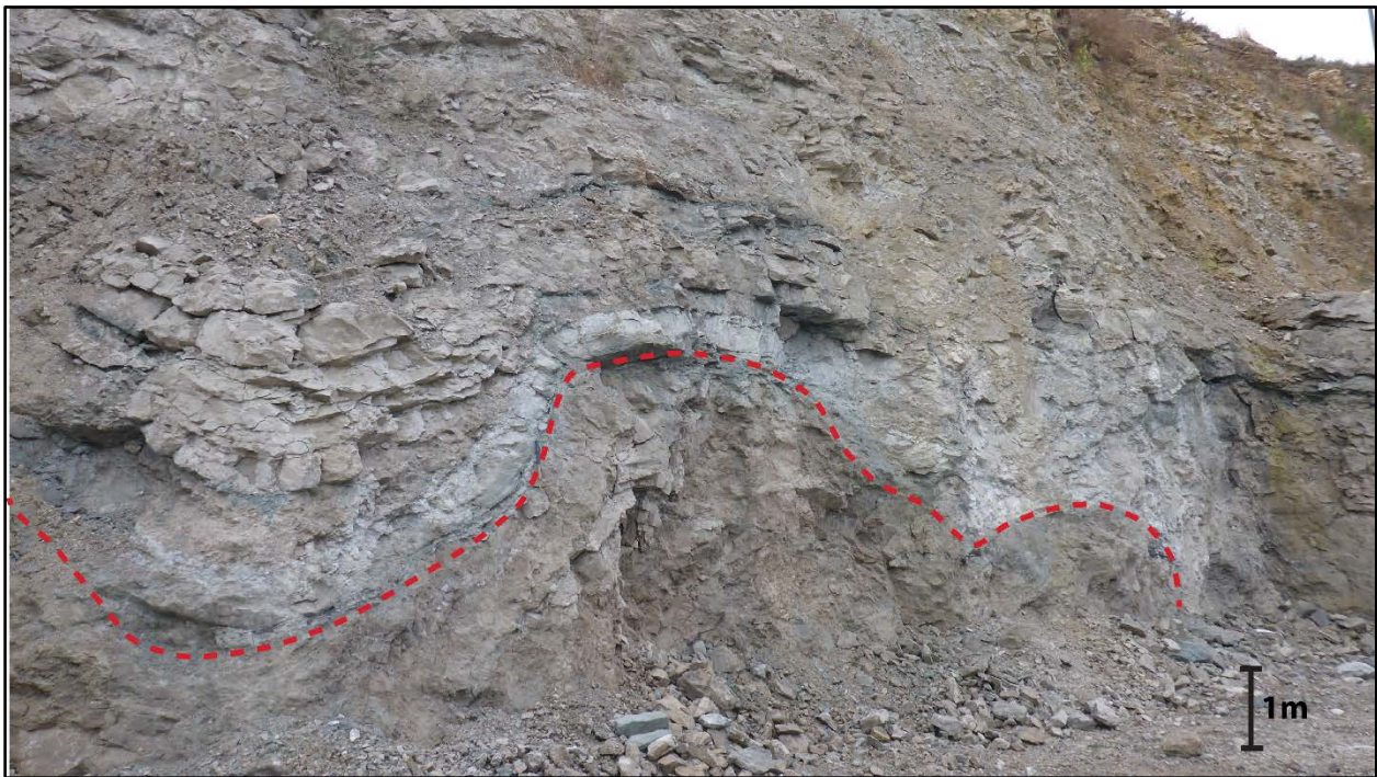
Figure 3: Disturbed bedding in the "St. Louis" Formation due to solution collapse seen in the Beach Quarry located in the extreme southeastern corner of the Salem Quadrangle. Basal dark brown dolomite is pervasively brecciated.
