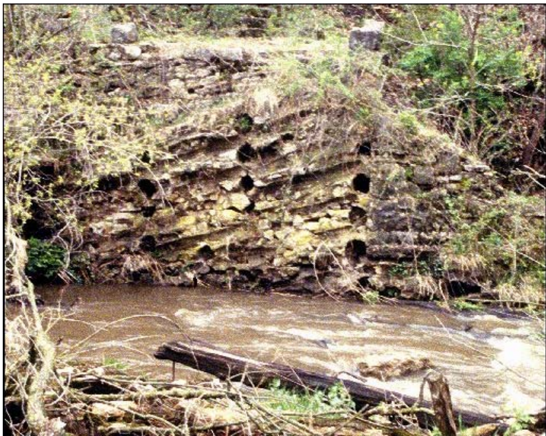
Figure 7. Old CCC dam structure on north bank of Otter Creek.
