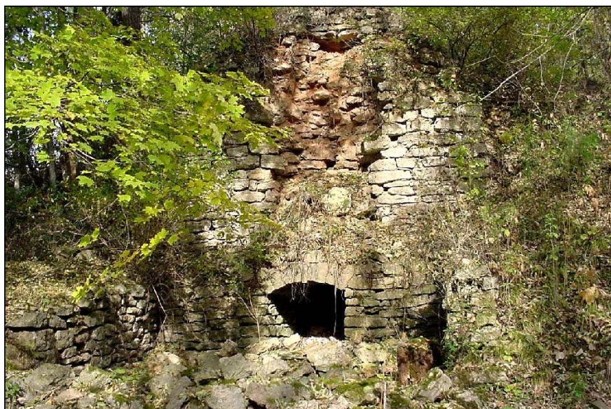
Figure 5. Photograph of the lime kiln at Echo Valley State Park.
