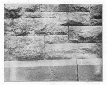
FIG. 100. Use of Galena dolomite in massive construction.
