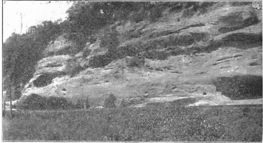
FIG. 69. Bluff of Coal Measure sandstone at Cliffland station, showing the massive character of the rock and the irregular way it weathers.
