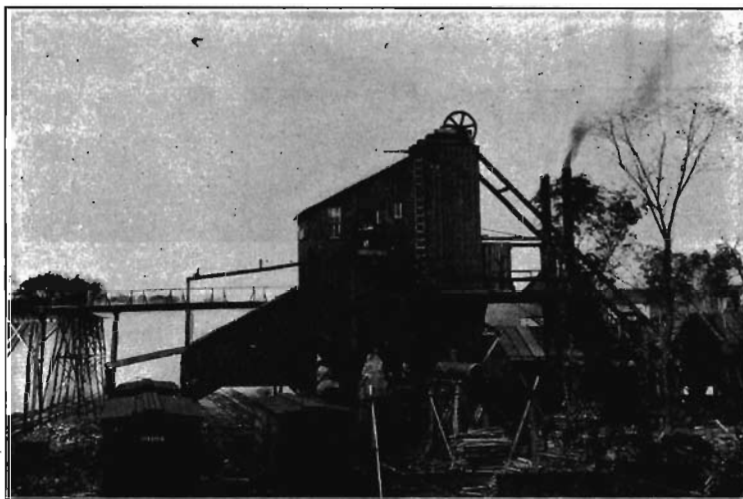
FIG. 64. Tipple of shaft No. 2, Hocking Coal Company, Hocking.
