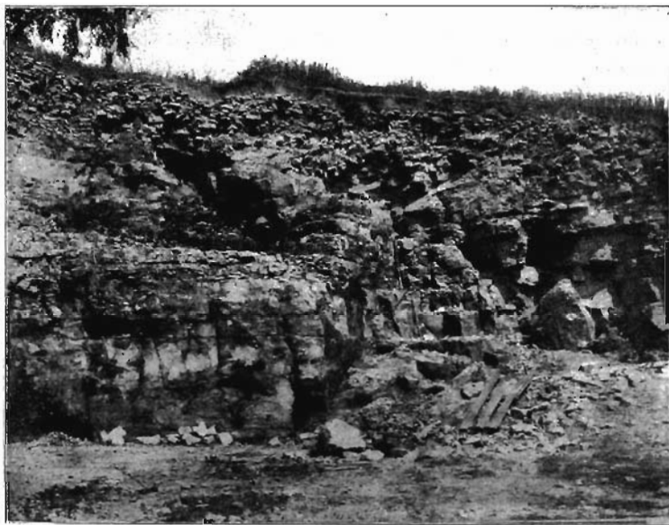
FIG. 35. Quarry in cherty dolomitic beds at the Gypidula comis horizon, a short distance above the bridge at Chickasaw.
