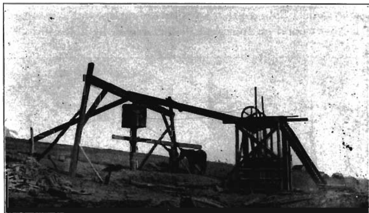
FIG. 61. Horse gin used in sinking a shaft near Foster.
