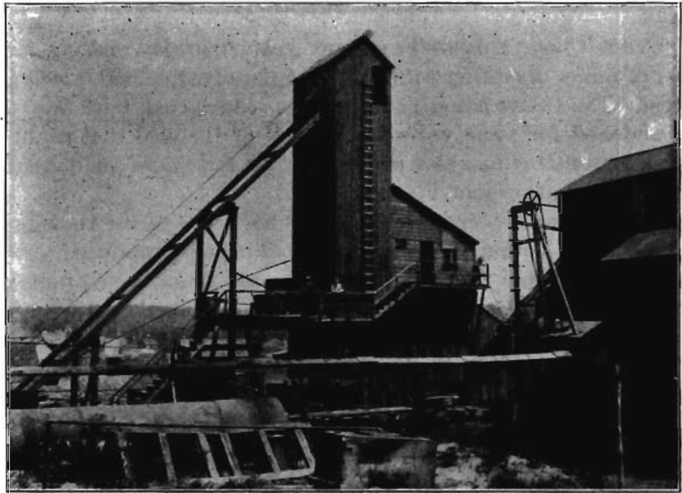
FIG. 63. Tippie and screening plant at shaft No. 1, Hocking Coal Company, Hocking.
