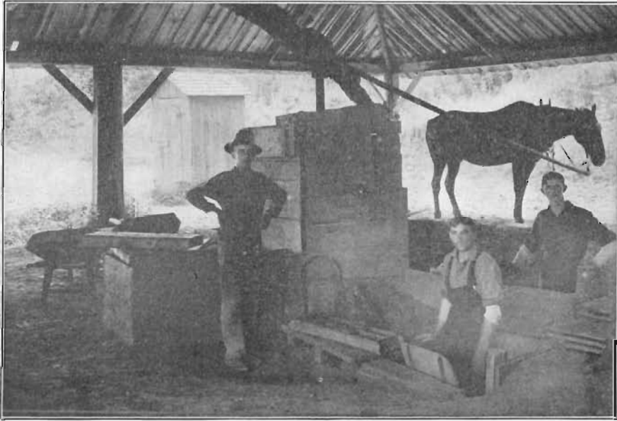
FIG. 75. Brick machine used in the manufacture of soft mud brick. William Samuels yard, Muscatine, Iowa.
