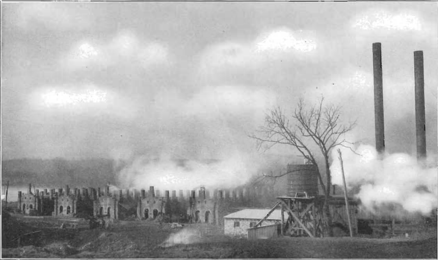
PLATE XXIV. Plant of the Flint Brick Company, Des Moines, Iowa.
