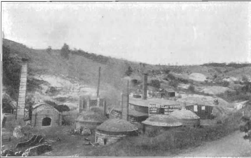
FIG. 47. Plant of the Boone Clay Works Boone, Iowa.
