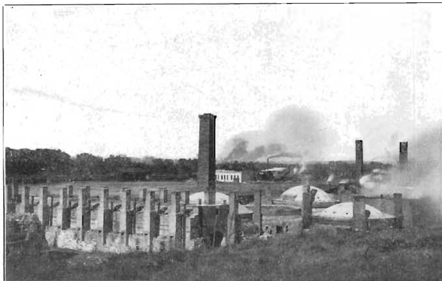
FIG. 56. A portion of the plant of the Merrill Brick Company, Des Moines, Iowa.
