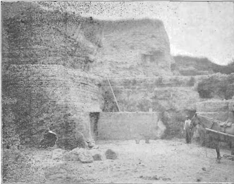
FIG. 50. Williams' quarry near the east side of section 24, Clermont township. The thick layers in the lower portion furnish the good stone.
