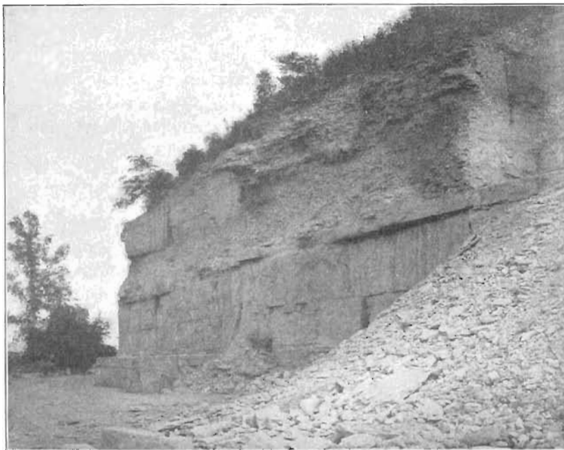
FIG. 9—Quarry in Lower Buff beds at McGregor. Thin-bedded limestone is seen at top.
