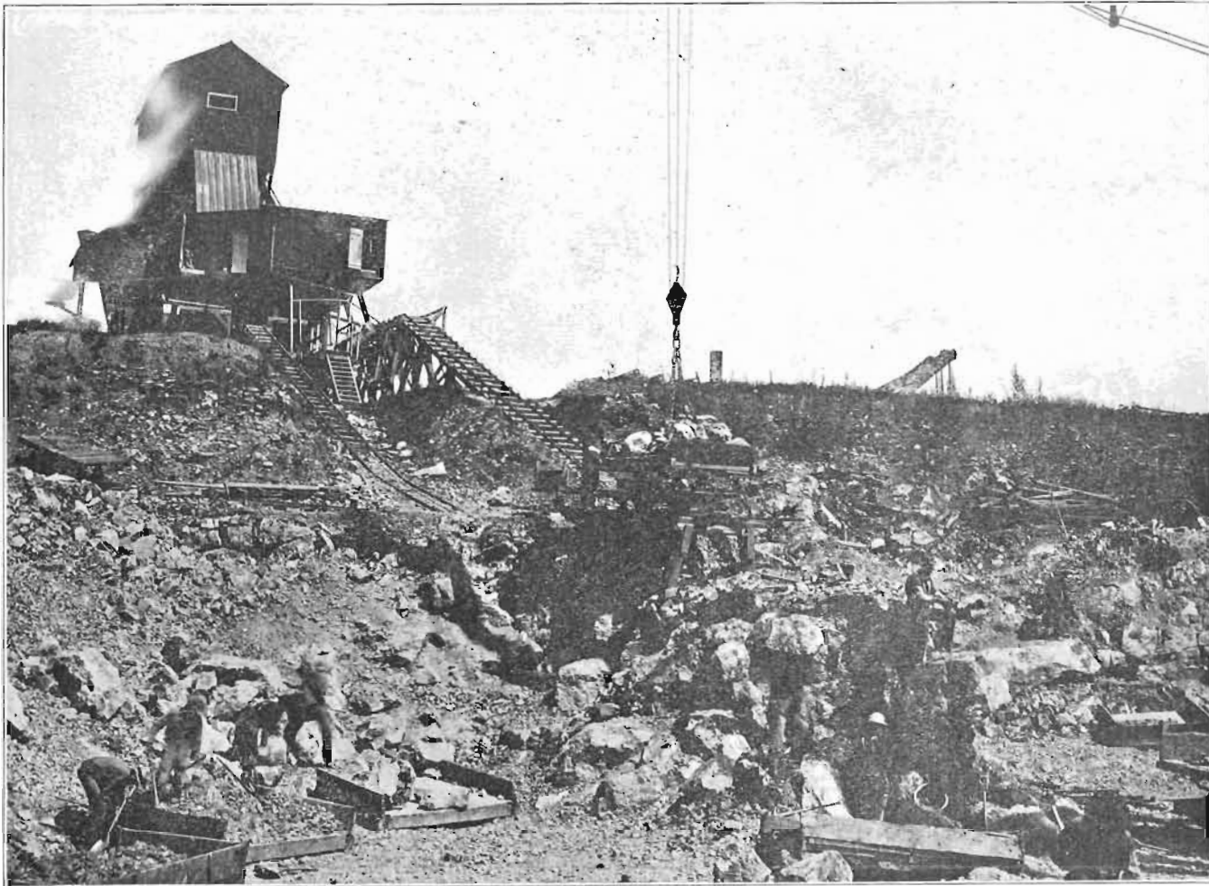
PLATE XLV—Quarry and crusher plant of Cedar River Stone Company, near Waverly, Bremer county, Iowa. The quarry stone is brought to a platform at foot of an inclined plane leading to crusher. The irregularly bedded stage of the Devenian is well shown in the quarry.
