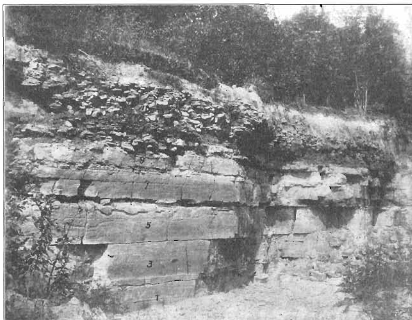
FIG. 27—The Lewis lime quarry, in the southeast quarter of section 27, Osage township, one and one-half miles southwest of Osage.
