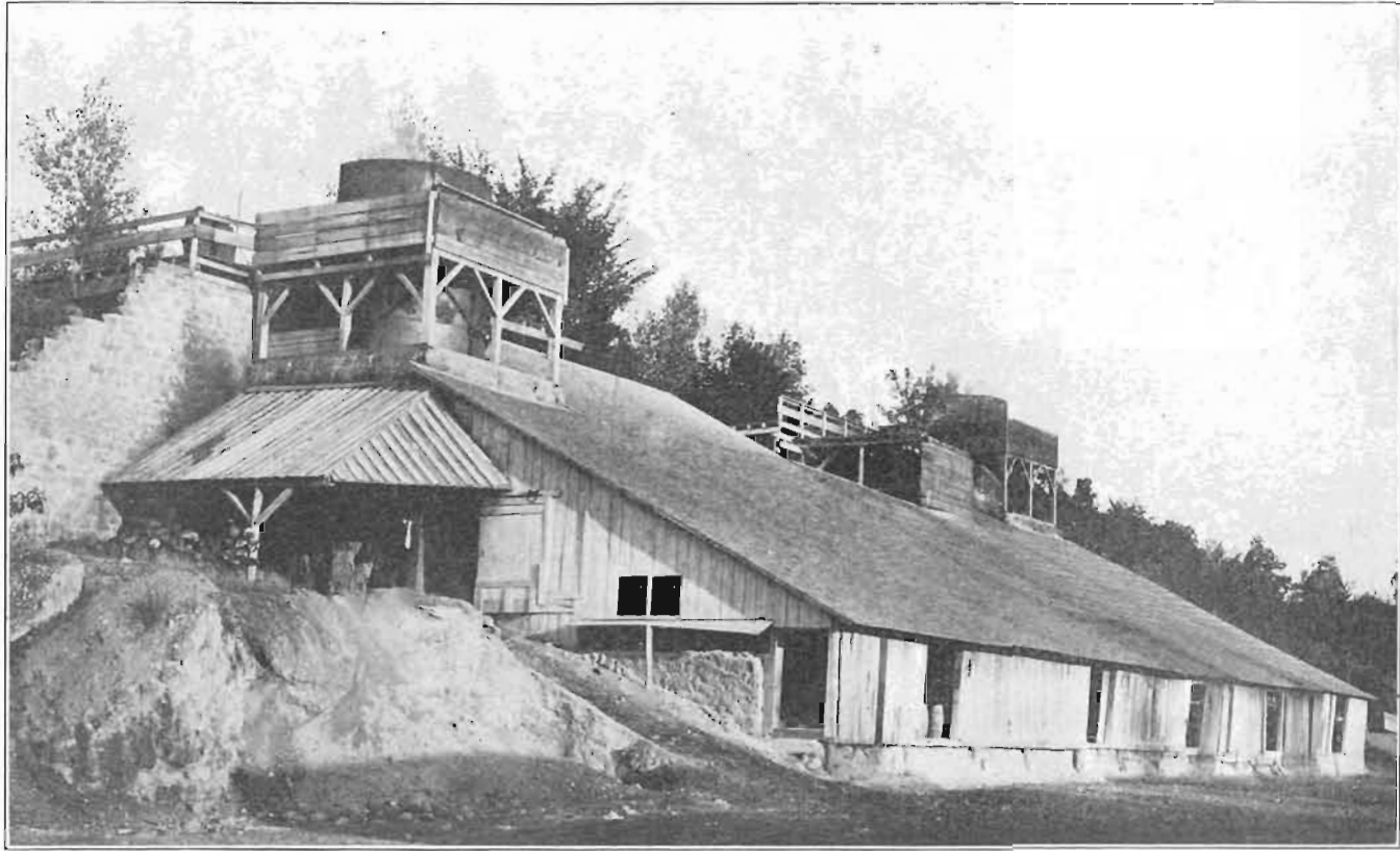
PLATE XL--A. Hurst Lime Company plant at Pinhook, showing elevated track, kilns and stock house. A fair representative of the lime manufacturing plants of the state. Jackson county, Iowa.
