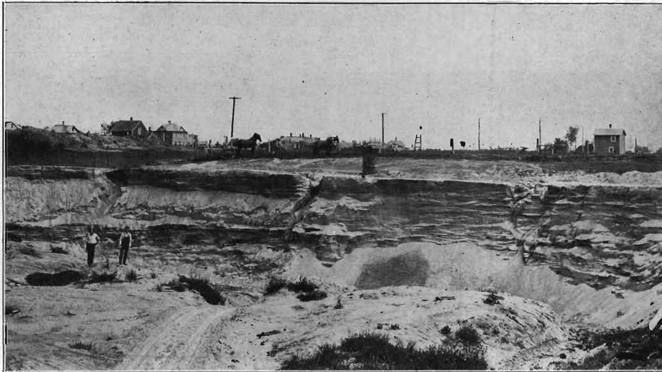
PLATE XXXI—The Miller-Montgomery pit showing pit methods. Doon, Lyon county.
