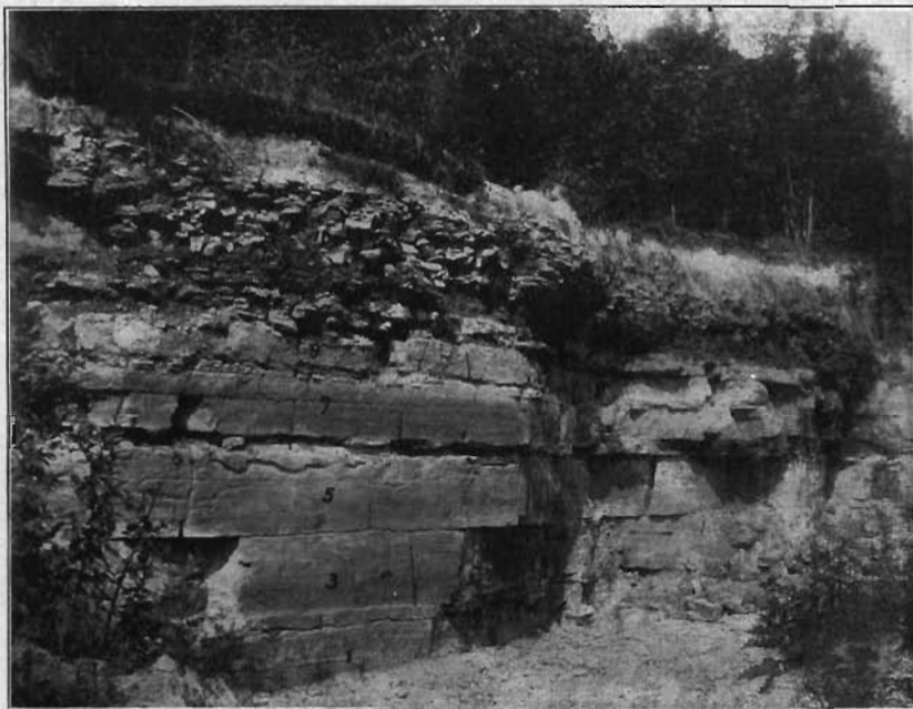
FIG. 51.—The Lewis lime quarry, in southeast quarter of section 27, Osage township, Mitchell county, one and one-half miles southwest of Osage. The beds exposed are hard and compact and are fairly representative of the vicinity.
