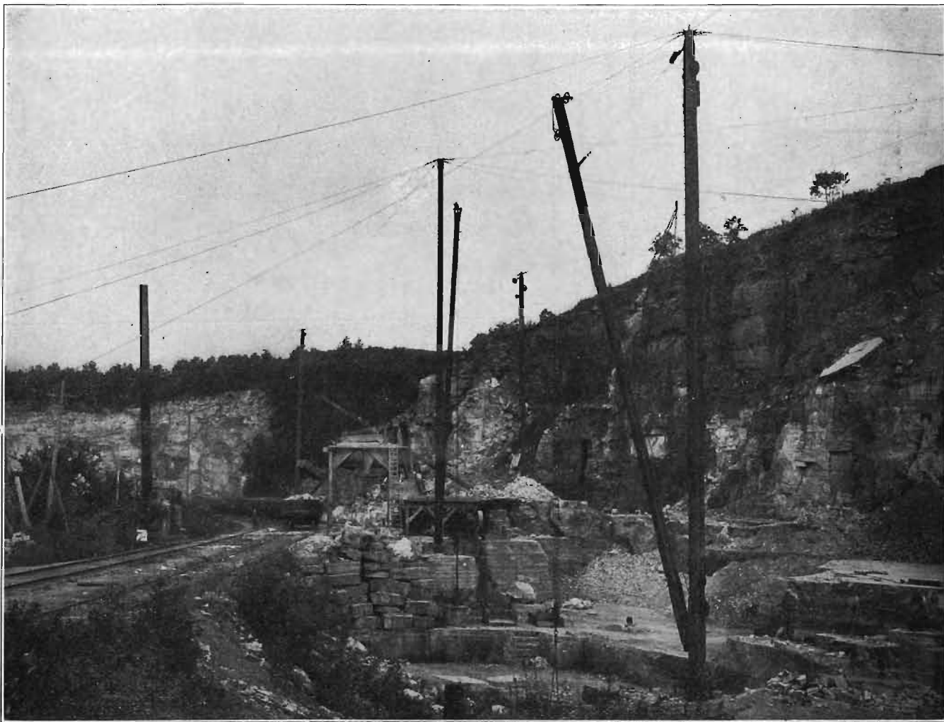
PLATE XXVI—John Ronen quarry, showing arrangement of tracks, derricks and crusher plant. Stone City, Jones county.
