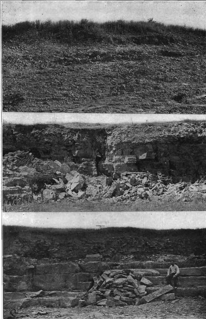
PLATE XXIII— a. City quarry about one and one-half miles north of Cresco. The product is a natural macadam. b. Quarry northeast of Elma showing flaggy character of beds. c. Hallman quarry showing principal quarry beds. Cresco, Howard county.
