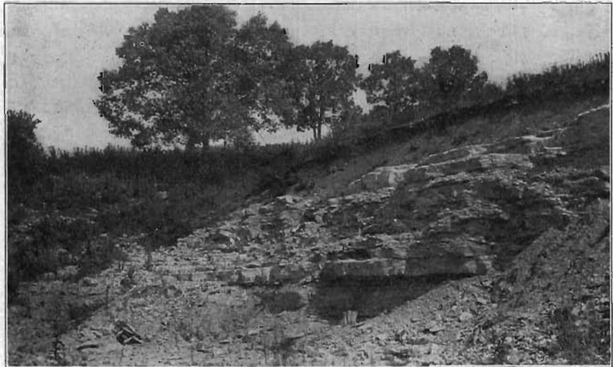
FIG. 46—Winterset quarry located about one-half mile southeast of the court house, Winterset, Madison county.
