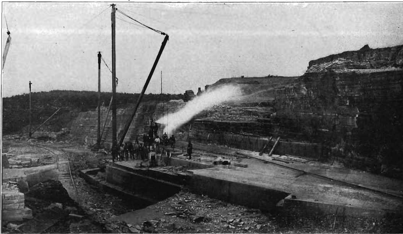
PLATE XXV—Champion quarry showing track and derrick arrangements and channeller. Stone City, Jones county. Crushed stone is the chief product at present.
