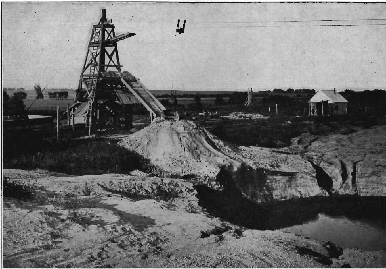
PLATE XLIV—Dalton pit showing aerial clam shell and loading chutes, LeMars, Plymouth county.
