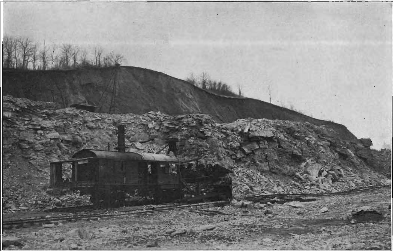
PLATE XXX—Quarry of the Chicago and North Western Railway, Cedar Rapids, showing steam shovel, drill rig and broken stone.
