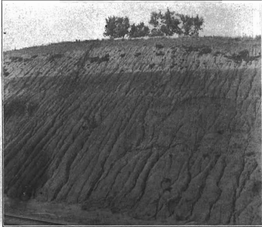
FIG. 21.—Railroad cut on Chicago, Milwaukee & St. Paul railway about two miles east of Dedham, Carroll county, Iowa. Cut shows loess, ferretto zone, and Kansan drift.
