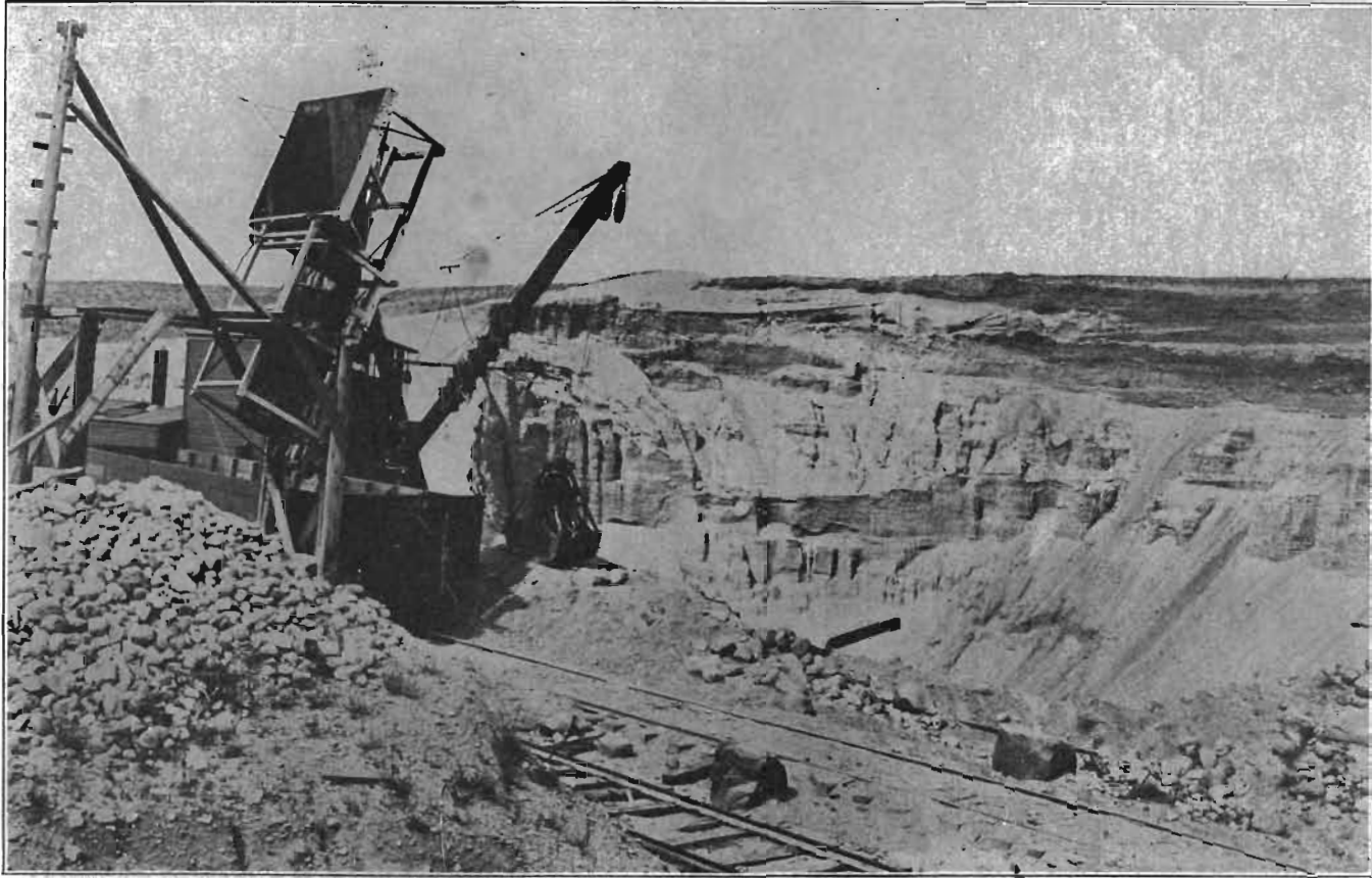
Gilleas pit in section 14, Cherokee township, Cherokee county. This is one of the largest exposures known in the region. The pit is worked by a steam clam-dipper to a depth of sixty feet below the terrace level. (Beyer, Iowa Geological Survey, volume XXIV, p. 157.)
