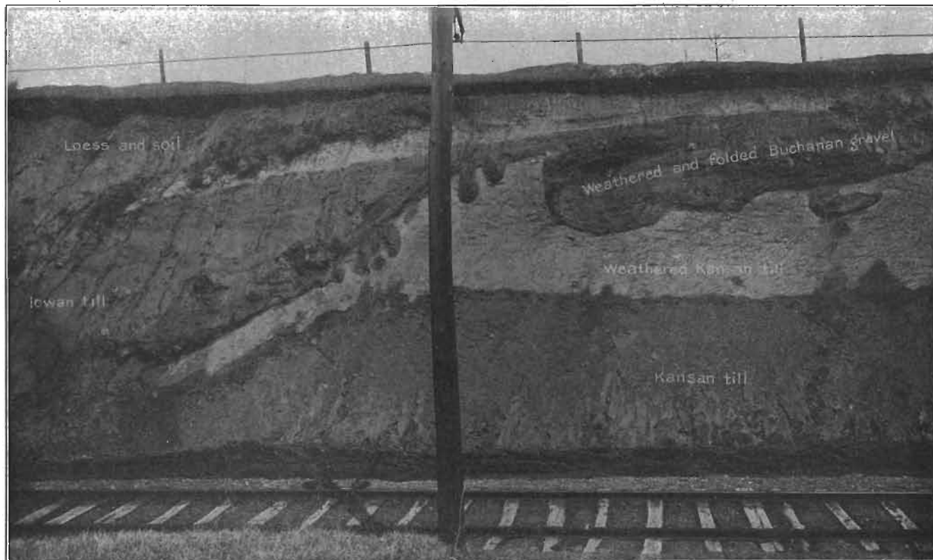
View of cut on interurban railway northwest of Iowa City, Iowa.
