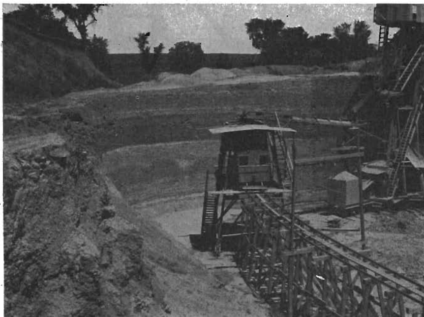
Figure 7. Shale pit of the United Brick and Tile Company, Adel, Dallas County, showing characteristic bedding of the Des Moines series.
