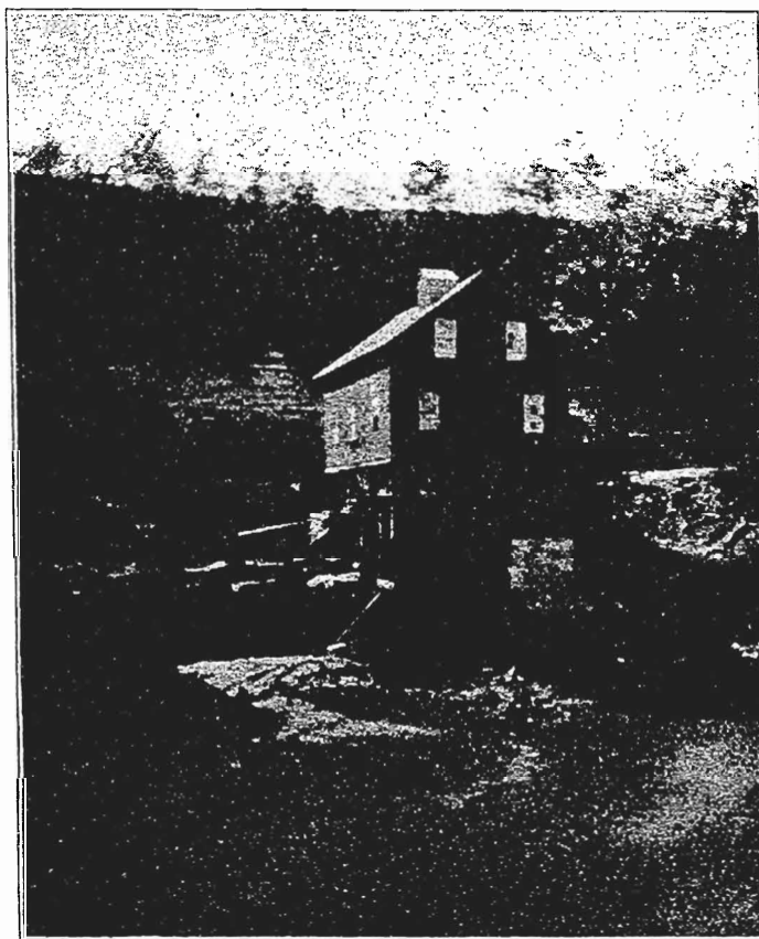
FIG. 76. The Tunnel mill at the Devil's Backbone. The main body of the limestone over the tunnel is the Earlham. That over which the water falls at the mill is the Fragmental.
