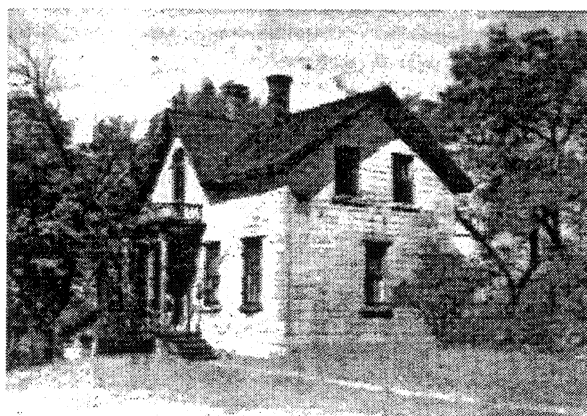
Figure 5. House in Fort Dodge constructed of gypsum blocks. All such houses have either been destroyed or the gypsum blocks have been covered by siding. No information is available about when the house was built. The image was scanned and computer enhanced from Wilder (1923, p. 201).
