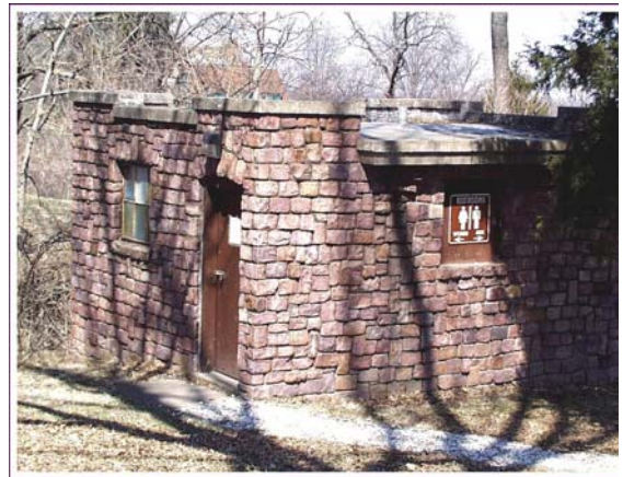
Figure 12, Restroom constructed of Baraboo Quartzite near Black Hawk Trail.
