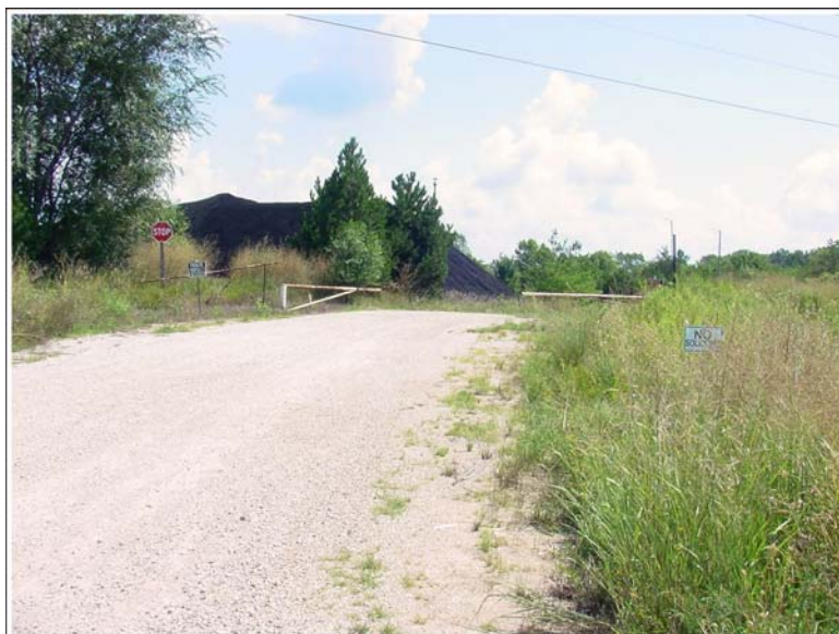
Figure 11. Entrance to Orba - Johnson Road.
