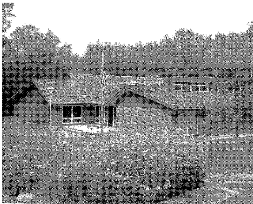
Figure 6. The office and classroom building at the Springbrook Conservation Education Center.
