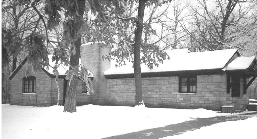
Figure 6. Pikes Peak's concession stand was constructed by the CCC in the 1930s.
