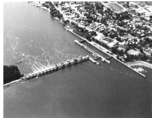
Figure 2. Lock and Dam 10 at Guttenburg
