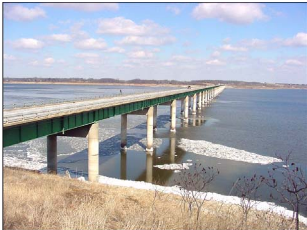
Figure 4. Photograph of the Highway 14 "mile-long bridge".
