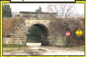
Ely St. Tunnel
