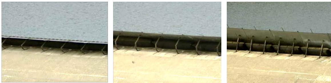
Figure 2. A sequence of photographs showing the raising of the pneumatic gates at the Saylorville Dam emergency spillway.
