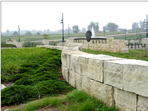
Figure 4. Anamosa Stone used in retaining wall construction at the Coral Ridge Mall, Coralville
