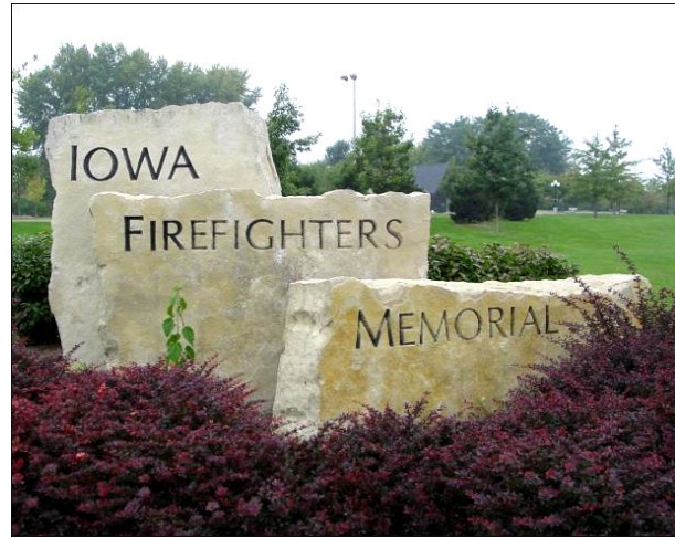
Figure 3. Anamosa Stone used for construction of the Iowa Firefighters Memorial in Coralville
