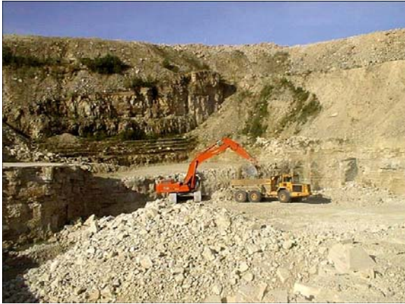
Figure 6. Unwanted overburden is removed from the rock ledge to be mined.
