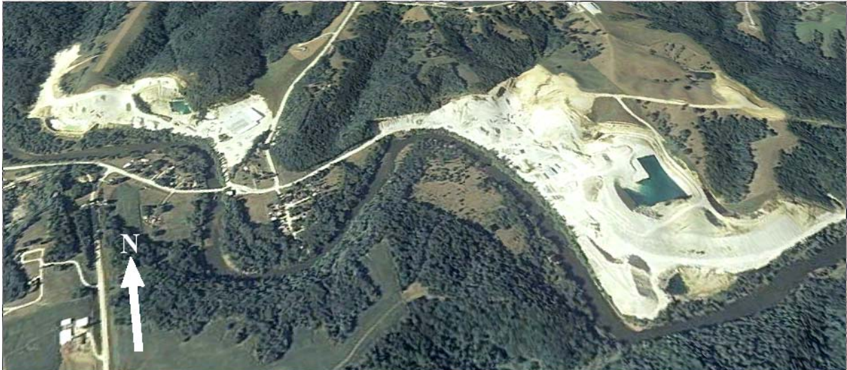
Figure 1. Oblique aerial photograph (looking north-northeast) of the Weber Stone Company quarries at
