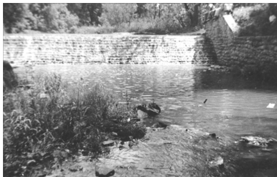
Figure 4. Swimming pool dam on Duchess Creek
