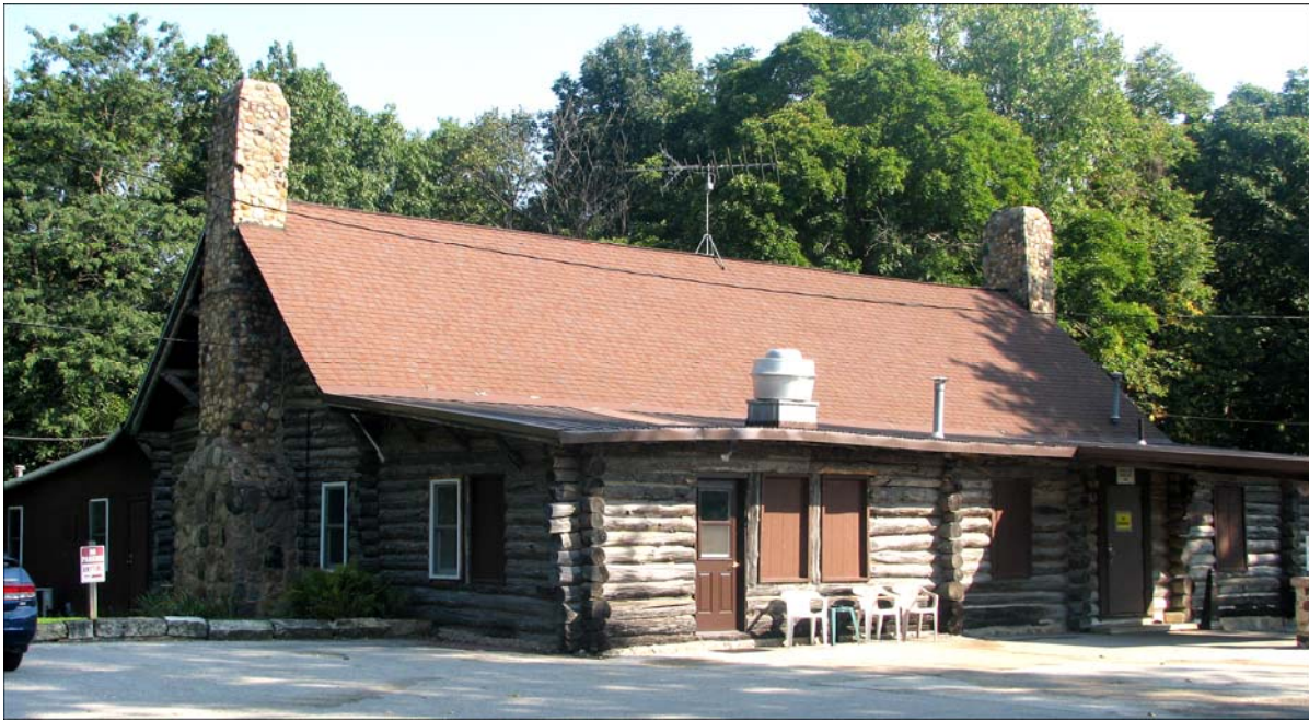
Figure 2. Clubhouse for the Wapsipinicon Golf Club at Wapsipinicon State Park, constructed in 1924.
