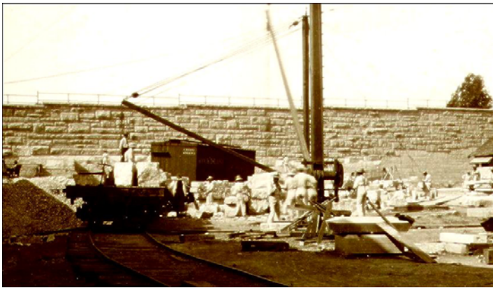
c. quarried stone being sized in the prison yard
