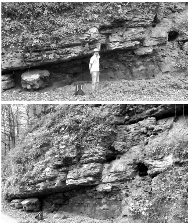
Figure 7. Two views of east dipping strata exposed along the road immediately south of the river, Wapsipinicon State Park (NE NW SW sec. 11). Evidence for dissolution of dolomite strata is evident by numerous vugs, pits, and small caves.
