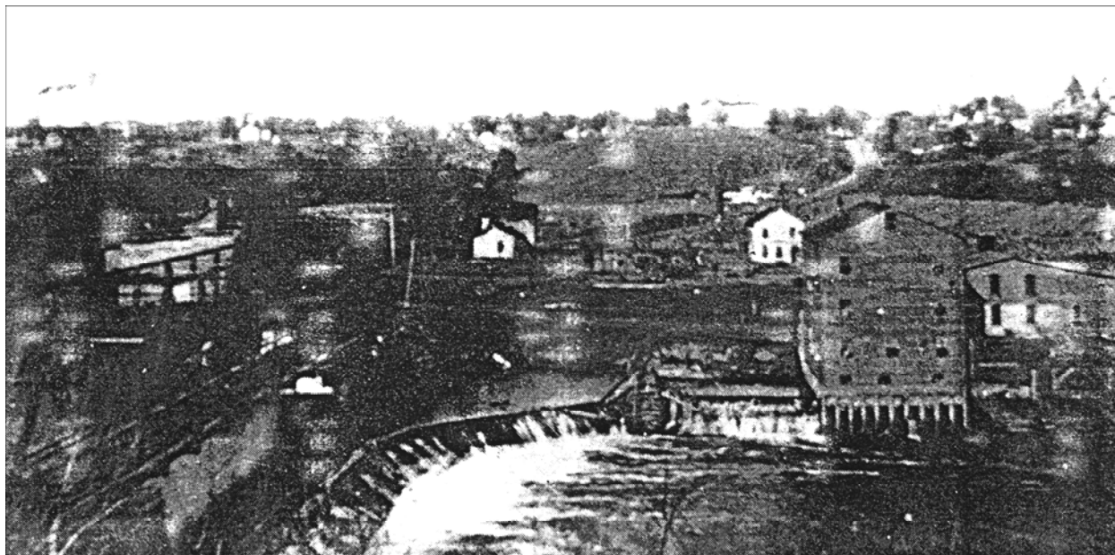
Figure 10. A view of Dillon's Bridge (left) and the old mill and dam on the north bank of the Wapsipinicon River. This late 1800s view (looking north from the rock bluffs in what is now Wapsipinicon State Park from a location very near field trip stop 8.
