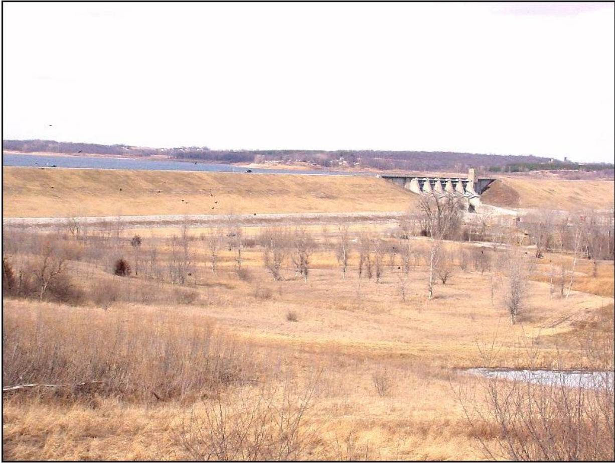
Figure 2. Photograph of the Red Rock Dam.
