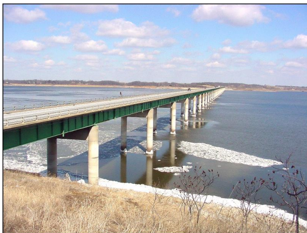
Figure 4. Photograph of the Highway 14 "mile-long bridge".
