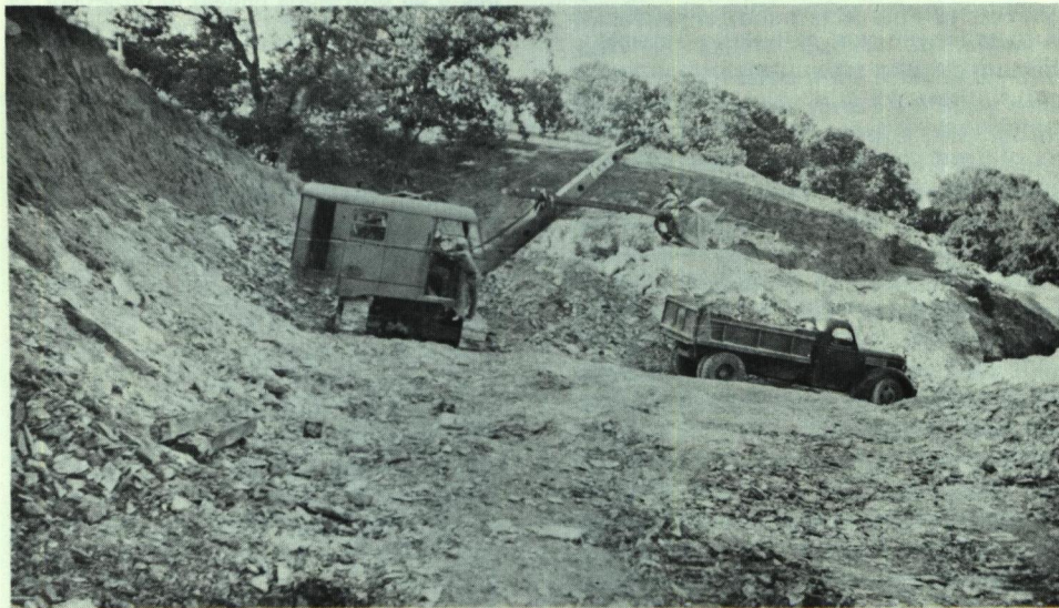
The Le Mars Quarry, owned by Fort Dodge Limestone Company, is shown during its first year of operation in 1948. The shovel and truck are used to excavate and haul the Cretaceous-age limestone to a nearby crusher.
