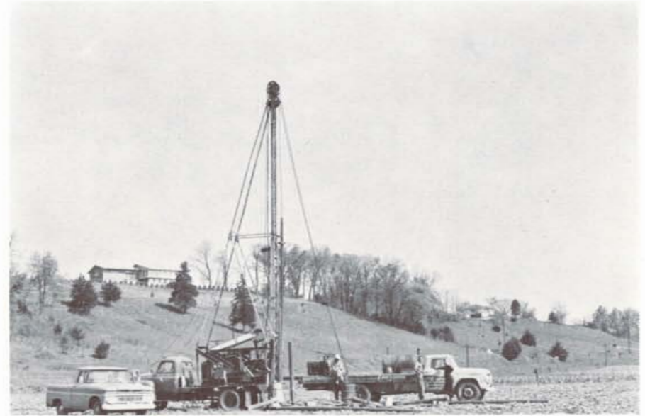
Water well being drilled into the alluvial aquifer of the Mississippi River Valley
