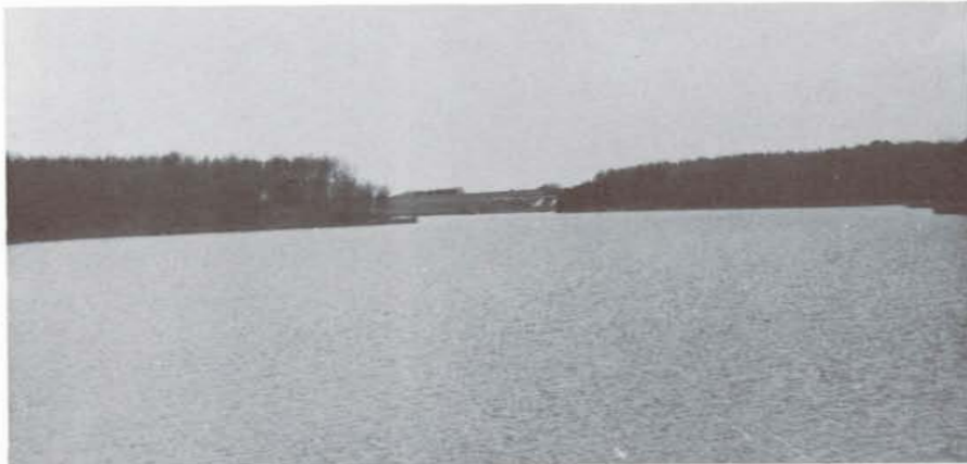
Corydon City Reservoir, Wayne County
