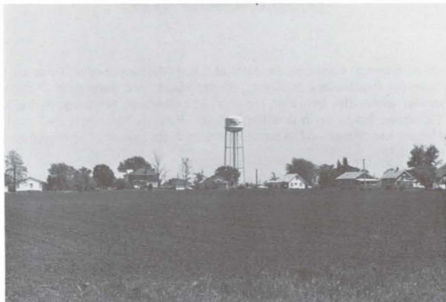
Rathbun Water Association water tower at Williamson, Lucas County
